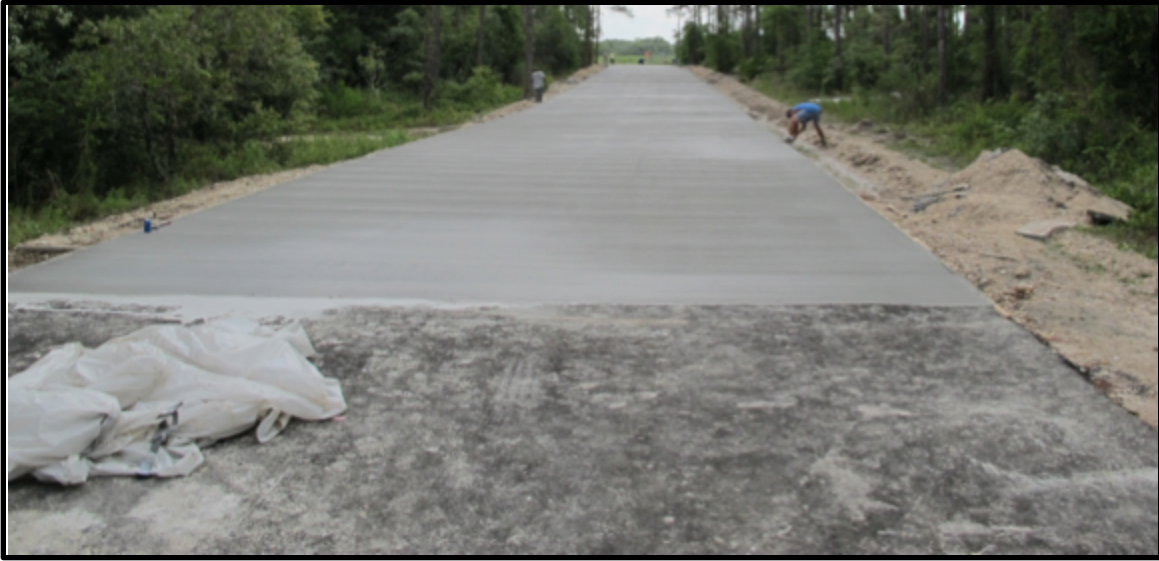
Figure 4. Final Touches Being Put On The Concrete Segment Of The Test Roadway
