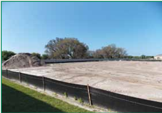
Silt Fence at Construction Site
