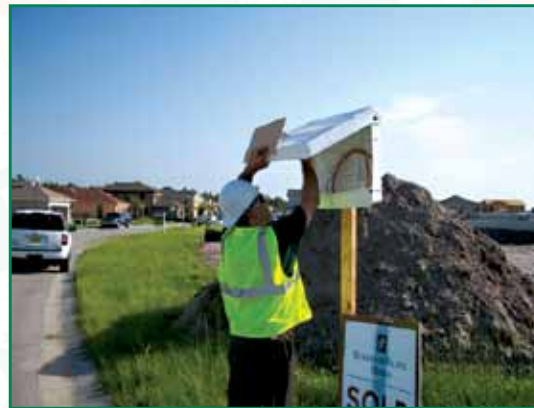
Construction Box with Plans
