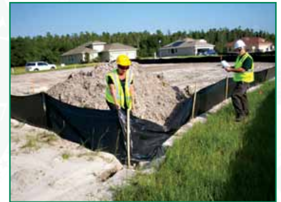
County Inspectors at Construction Site
